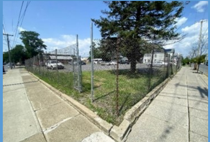
City owned lot at the corner of N. 4th Street and State Street slated to be developed for affordable housing.
